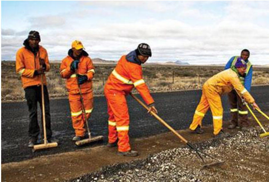
EMPLOYMENT: A tar road being laid between Warden and Standerton will link with Gauteng, Mpumalanga and KwaZulu-Natal. Internal streets in Vrede are currently being used as bypasses. PICTURE: GALLO IMAGES
