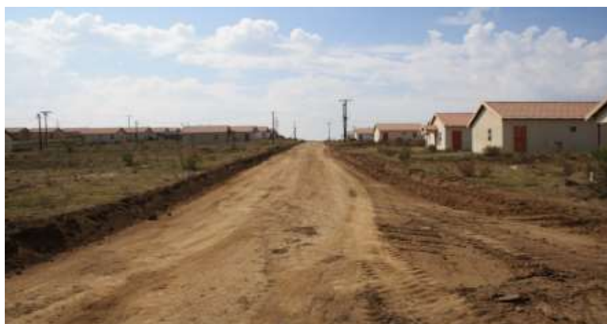
New roads under construction in Thembalihle Extension4
